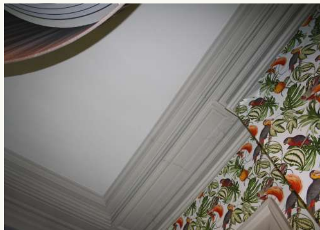
scheuren in molures
